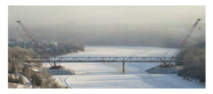
More than 10m tall access berm design in downtown Edmonton for old bridge removal and new bridge installation over the North Saskatchewan River. Extremely tight displacement requirements along with restricted type of material use for 100T crawler cranes. Possible high water level fluctuations, different types of crane, partial removal of the berm for cofferdam installation was among the variables
